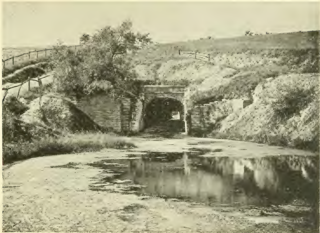
OLDEST TUNNEL IN THE UNITED STATES, BUILT 1825 FOR UNION CANAL—730 FEET LONG.
